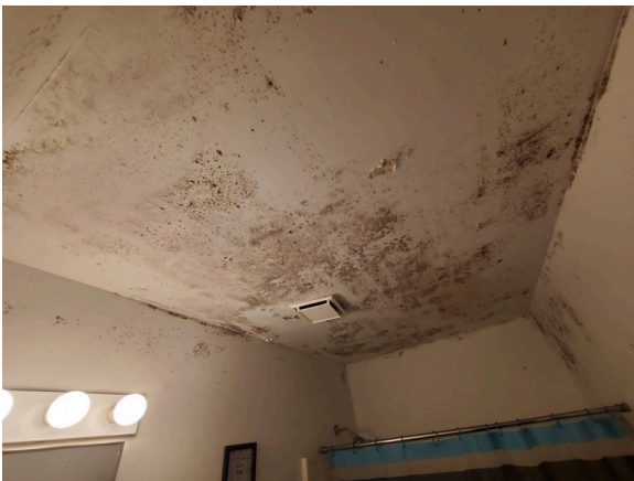
Mildew growth in bathroom of F4
