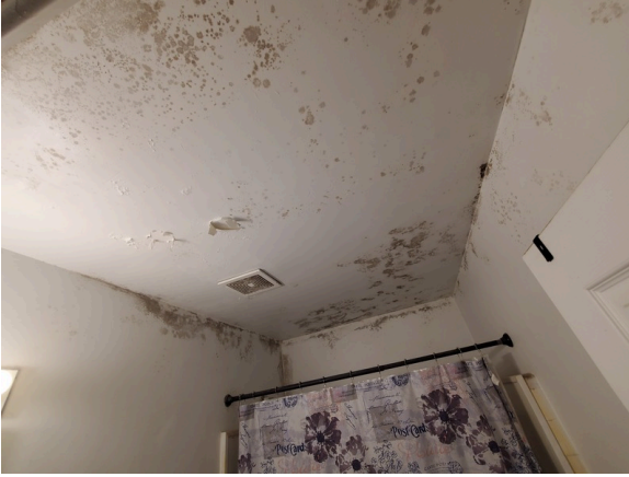
Microbial growth in bathroom of E3
