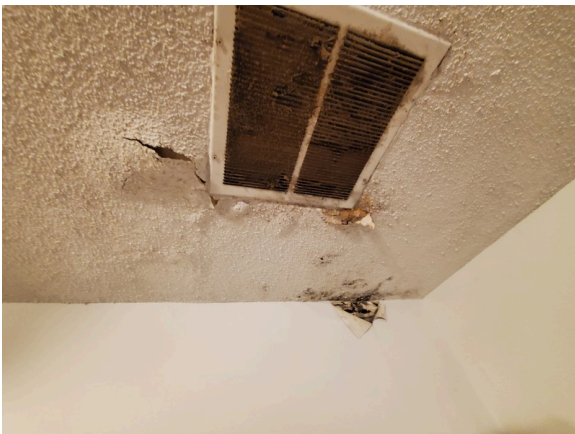
Water damage around return at H4
